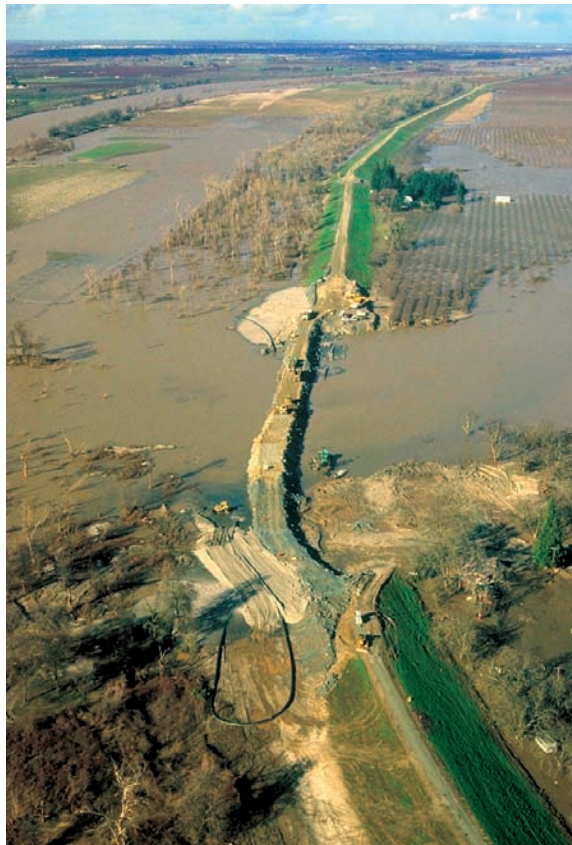
A breached levee along the Sacramento River, California, is being repaired.
