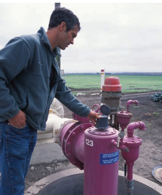
An extension specialist examines a purple pipe used for wastewater irrigation.
