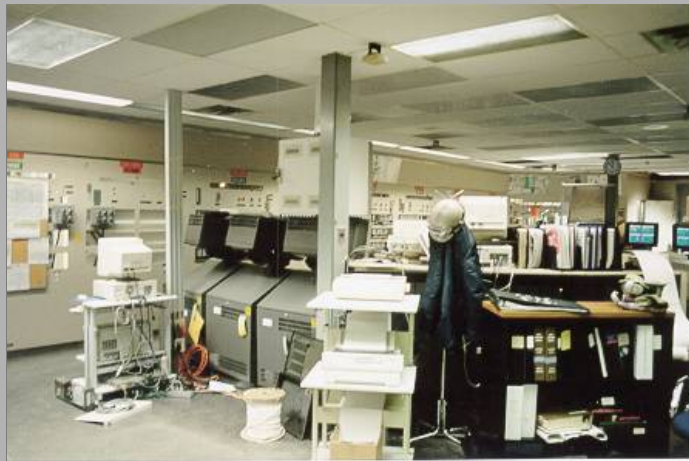
Control Room -- Before
